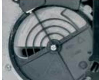
Air damper partially open (GS3, GS5)
